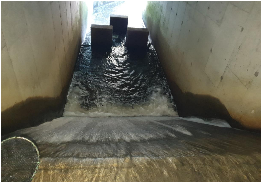
Figur 14: Vandringshinder under Vikhammerdalen.
