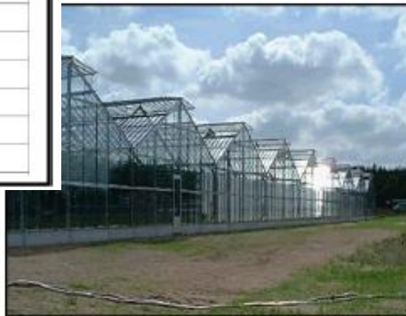
Fig. 3 A high-end closed bioreactor system. The worlds largest closed photo-bioreactor in Klötze, near Wolfsburg, Germany (Bioprodukte Prof. Steinberg; www.algamed.de ); the 700 m 3 are distributed in 500 km of tubes and produce up to 100 t algae biomass per year
