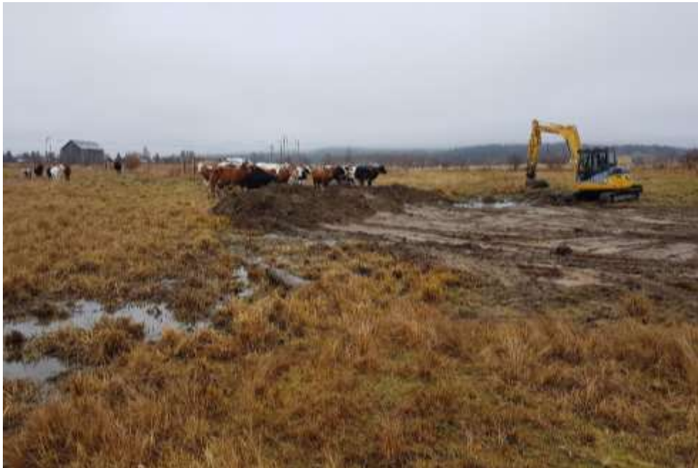
Filling of a ditch on a Northern pasture
